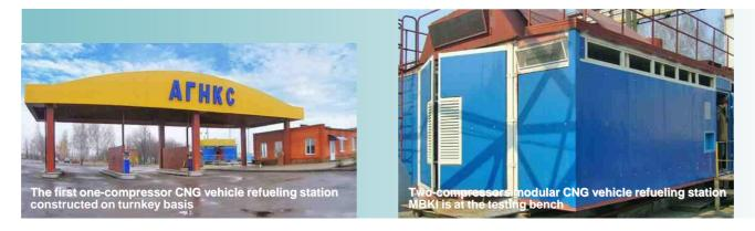
Process equipment of one-and two-compressors modular CNG vehicle refueling stations are operated in climatic zones with ambient temperature from -50°C to +45°C and in regions with seismicity up to 6 on the Richterscale.
